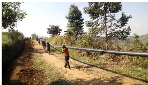
Carrying pipes in Kabere
