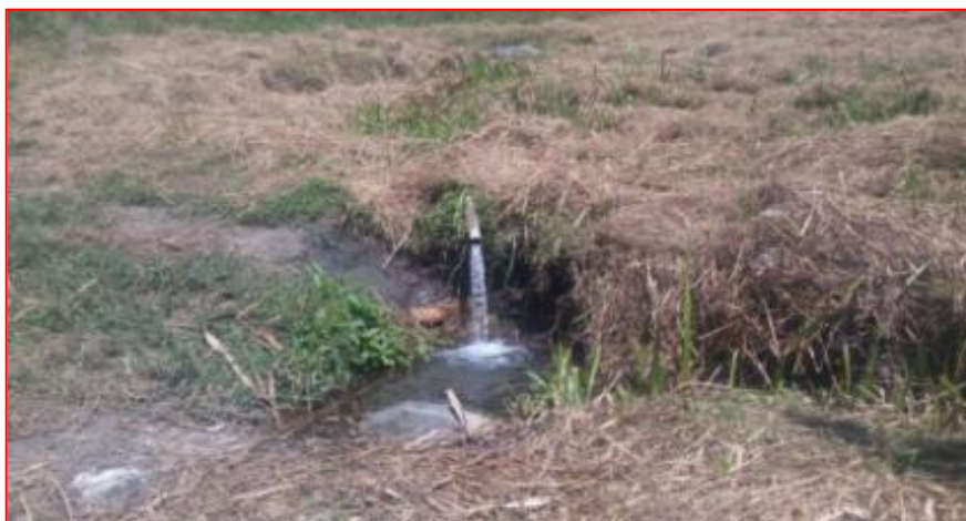
Source collection works for gravity adduction.
